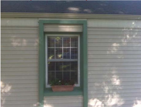
Repaired window trim pictured below
