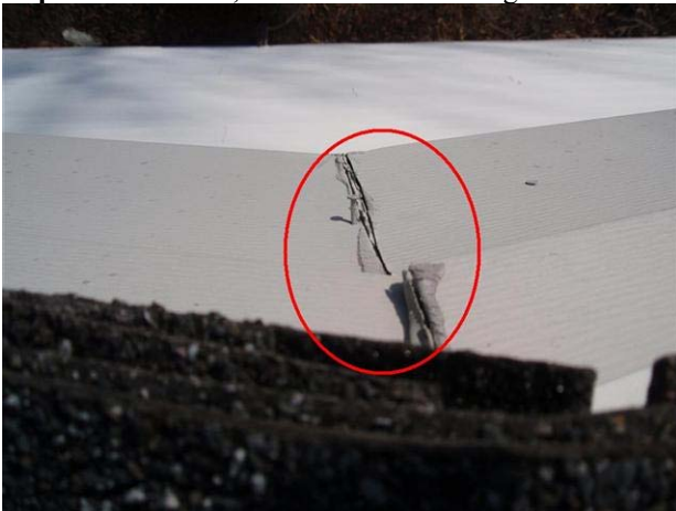
View from east roof ridge
